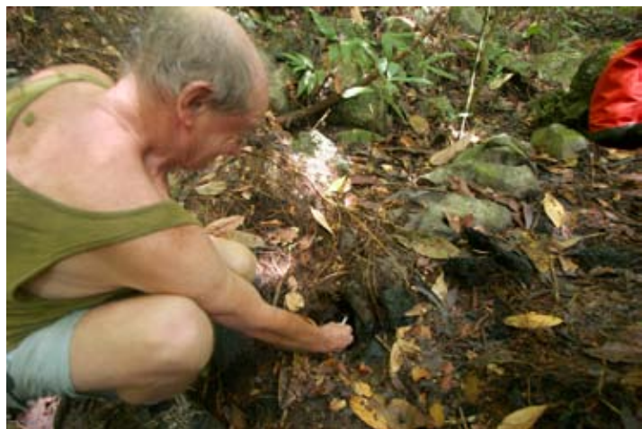
Smoke testing the draughting hole in the dry valley
